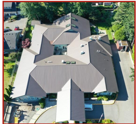
New metal roof is complete!
