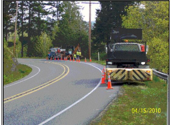
When a representative from DOT advised they were going to install more guardrails near Deception Café, we decided to pothole the fragile 10" AC pipeline to ensure that pipes would not be damaged again. Better safe than sorry I always say.
